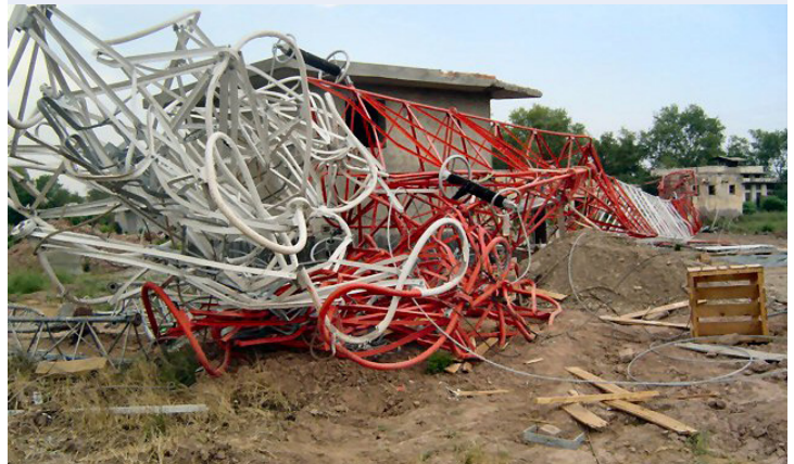
Radio Tower Collapse
