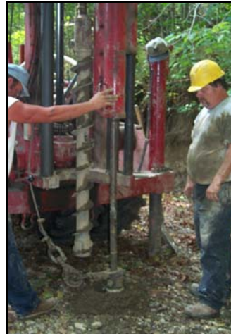
Drilling in Rugged Terrain
