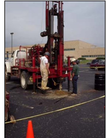
Drilling on Flat Terrain
