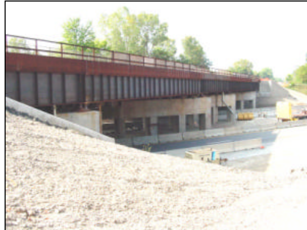
CSX Railroad Bridge over the Ohio Turnpike
